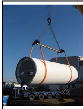
First shipment of steel arrives for the Margaret Hunt Hill Bridge
